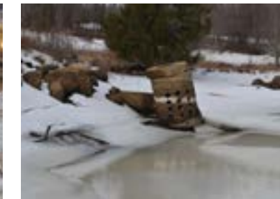
Fire suppression intake tower
