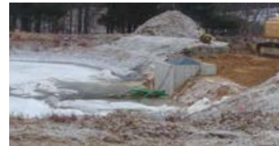
Drop inlet structure for controlling water level
