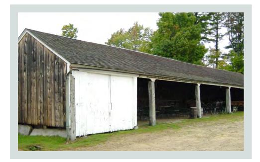
Located just east of the schoolhouse is this 110 x 25 feet structure constructed of vertical planks with a granite foundation and granite posts supporting the gable roof. The north end of the shed was primarily used as an ice house and the center for the storage of farm wagons. The Cart Shed was extensively rebuilt after the roof collapsed in the winter of 1982-83.
